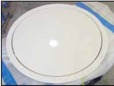
Escape hatch lift-out, Exterior view
