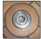
Bi-square, Installed flush with teak deck
