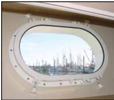
Oval portlight, Installed
